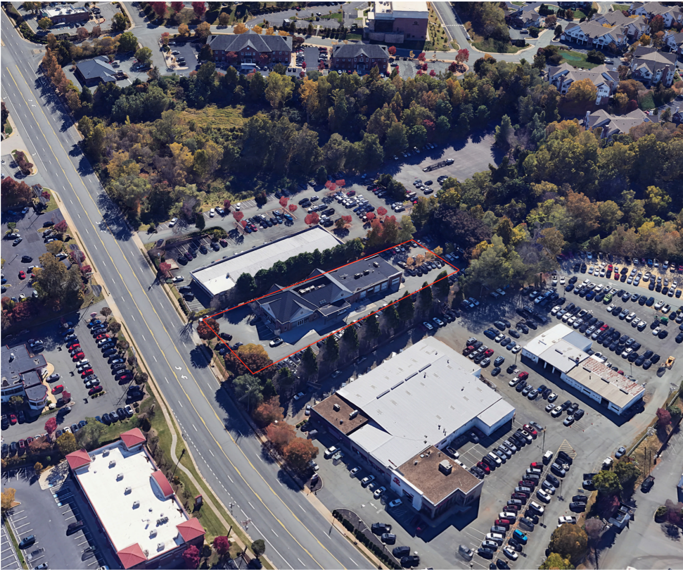
View from Richmond Rd
