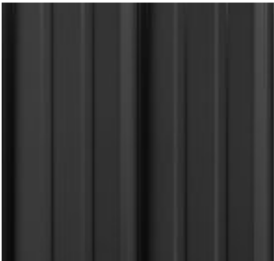
Roof Finish: Existing dark standing-seam metal roof, retained
